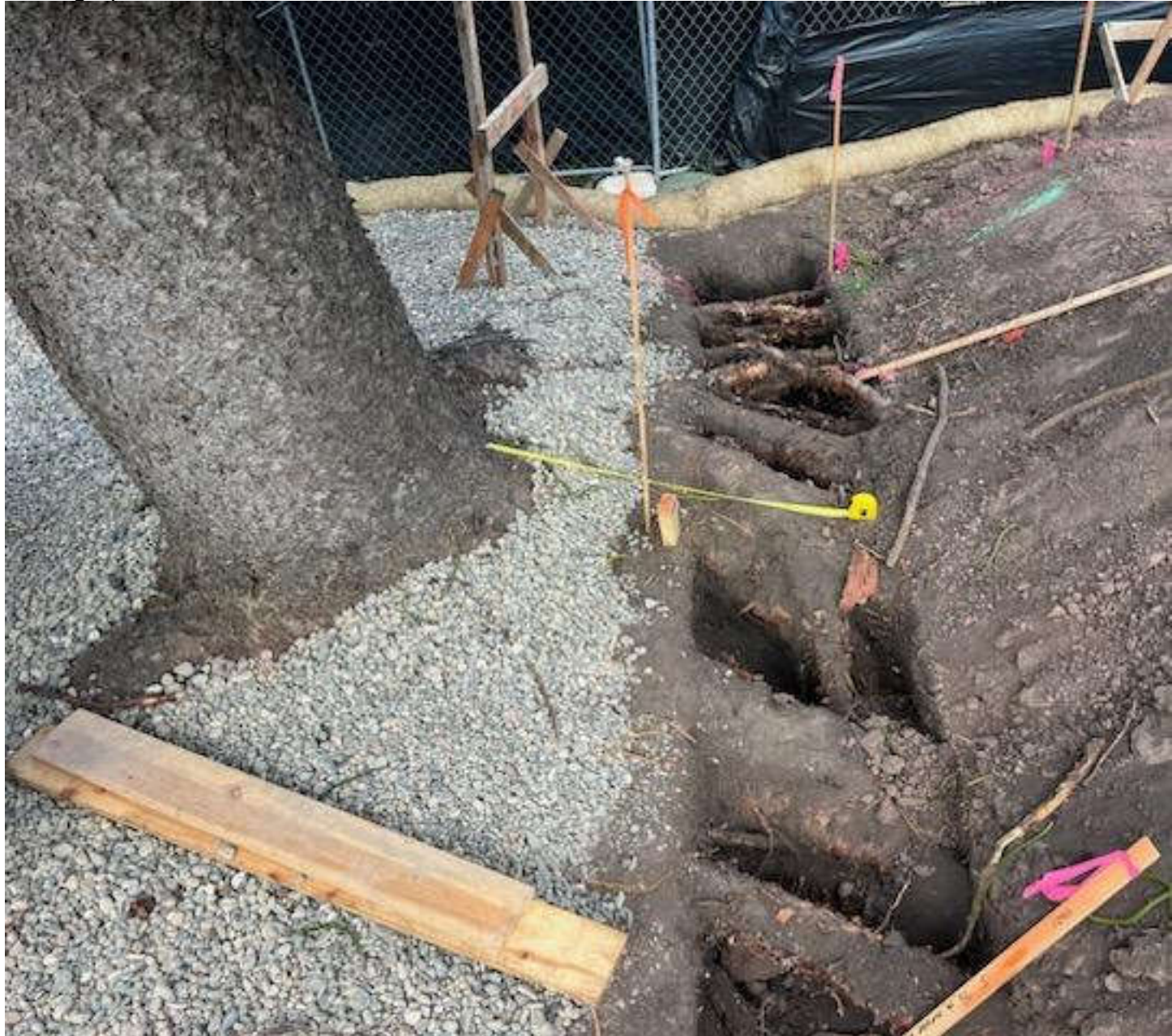
Photograph of Tree and Patio Foundation Trench
